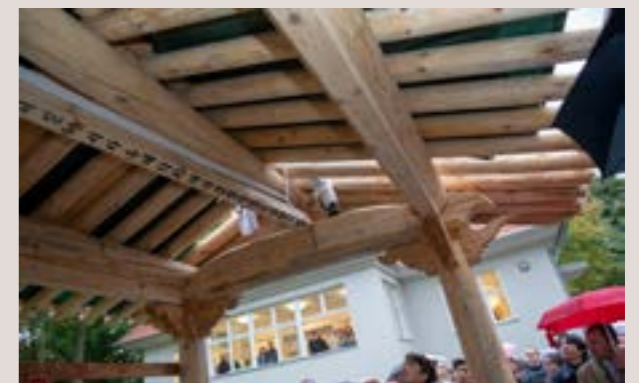
Raising the pavilion's ridge beam, October 2018
